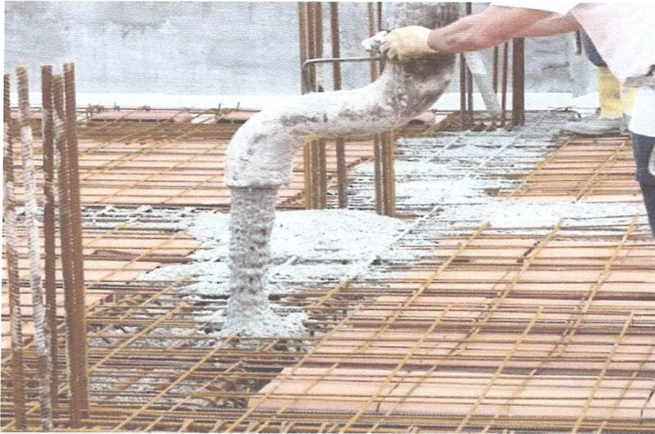
Figure III. 1 coulage d'une dalle
