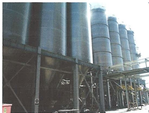
Figure II.15 : Silos de stockage [17].
