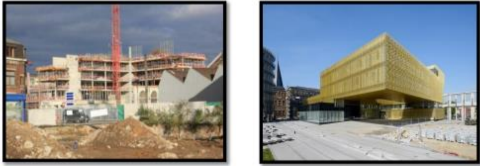
Figure 25 : Centre CIM chantier
