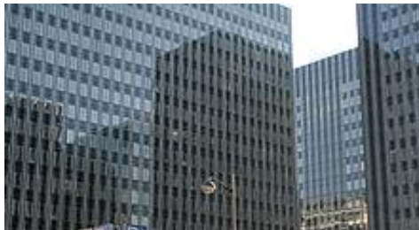
Figure 20 Curtain wall in Paris
