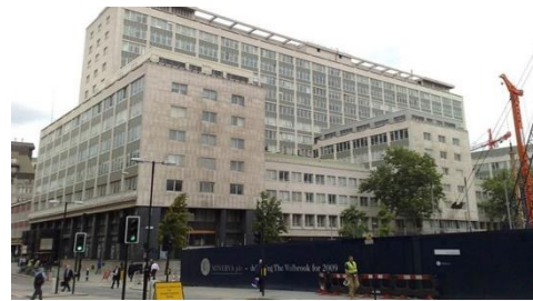
Figure 95 Bucklers bury house stood on the Bloomberg site before its demolition 2010
