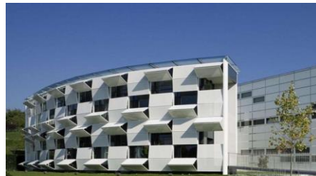
Figure 26 The dynamic solar shading of Kiefer Technic Showroom ( http://www.designindaba.com )
