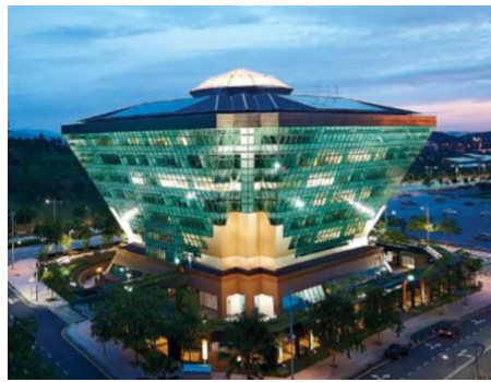
Figure 99 Energy Commission Diamond Building
