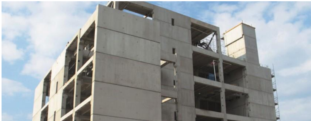
Figure 29 Precast concrete panels as shear walls ( http://www.esolution-pt.com )
