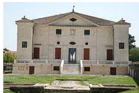
Figure 1.b Rear facade of Villa Caldogno
