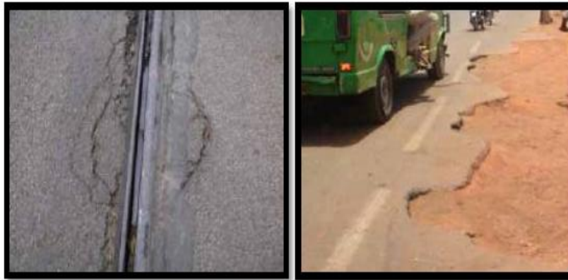
Fig.III.13: Epaufrures
