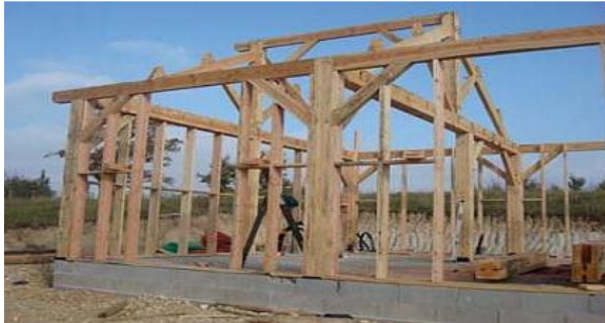
Figure 3-18 : Construction poteaux poutres
