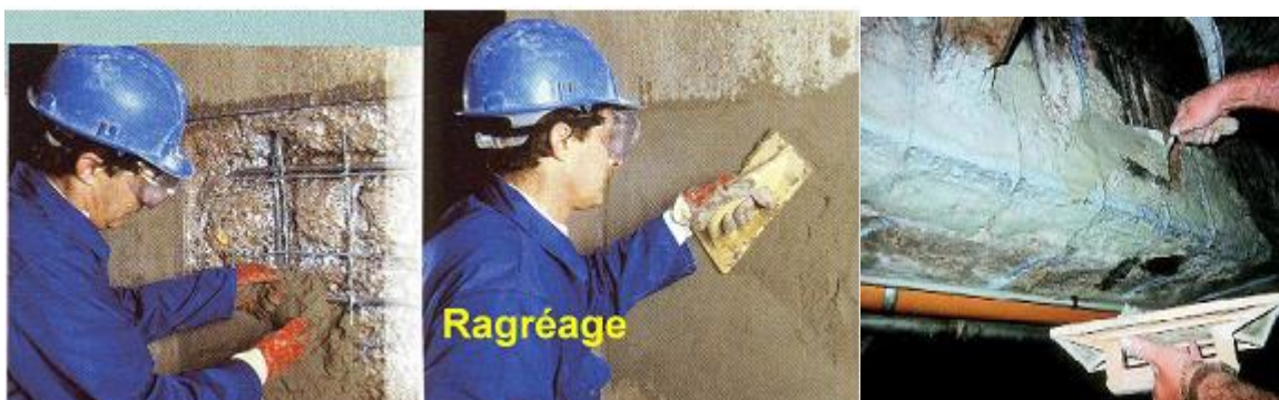
Figure III.3 : Application manuelle de mortiers
