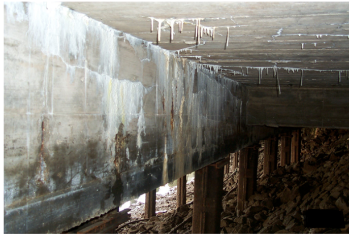
Figure I.6. Efflorescence du béton [THA-11].
