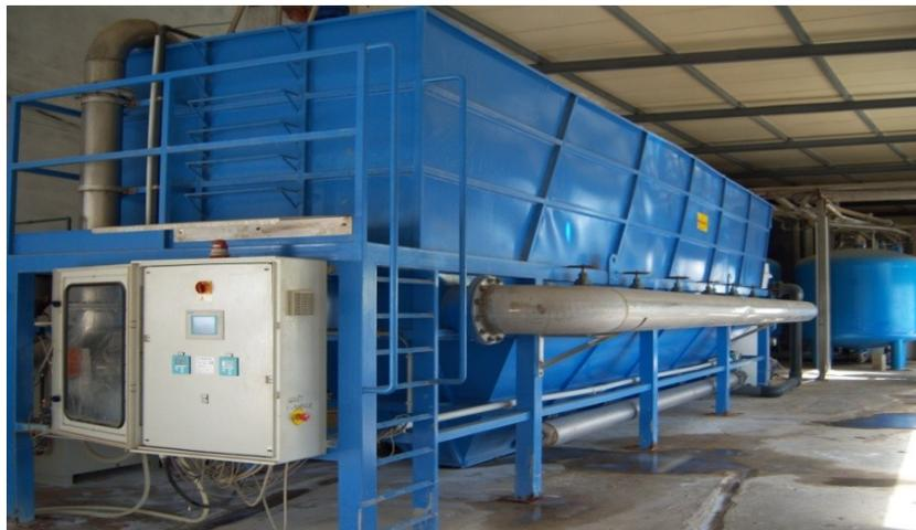
**Figure 07:** Bassin de la floculation- coagulation (CAB, 2013).
