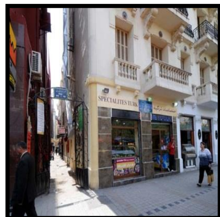
Figure10 façade d avenue H-B
