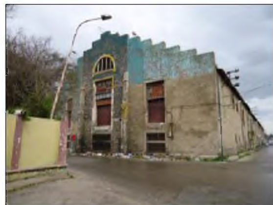
Figure 56: Dock n°4 Façade secondaire
