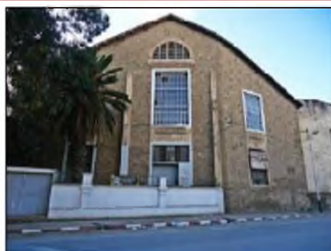
Figure 45: la façade principale
