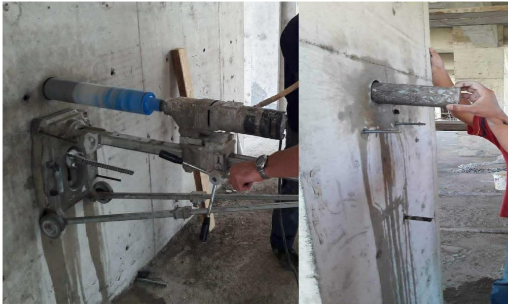
Fig 3.8. Core drilling in reinforced concrete for material sampling and inspection.
