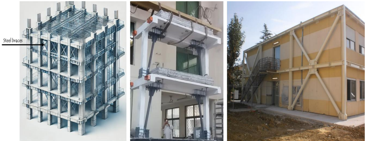
Fig 2.12. RC Building with Added Steel Braces for Enhanced Seismic Load Path and Stiffness [8].
