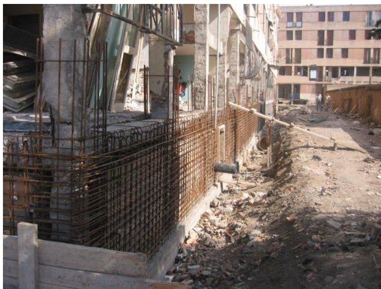
Fig 2.13. Reinforced Concrete Building with Added Shear Walls [8].
