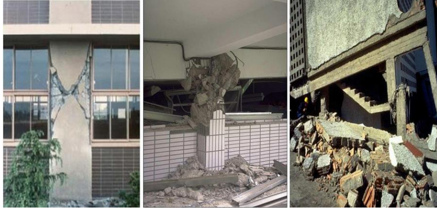
Fig 3.10. Vulnerability of short columns under seismic loading.
