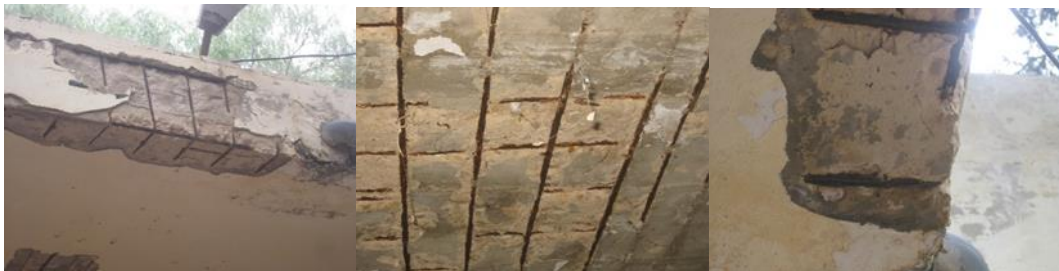
Fig 2.5. Reinforcement Corrosion.
