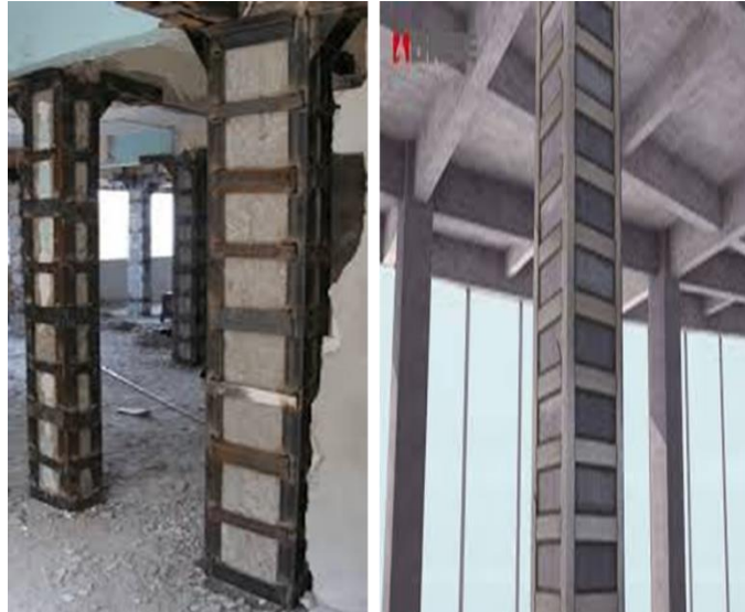
Fig 2.11. Reinforced Concrete Column with Steel Jacket [8].
