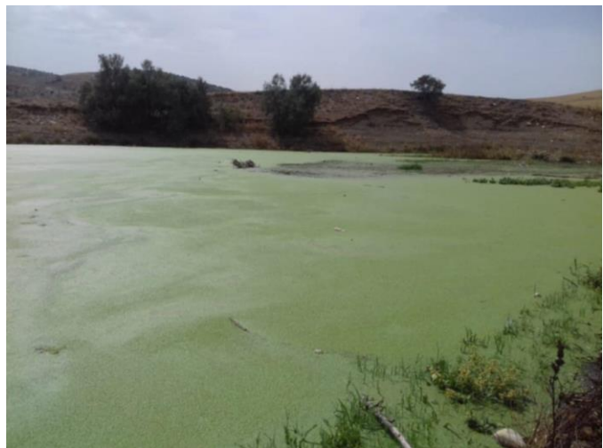
Figure 17: Medjez el Bgare dam (Gharbi,2023).
