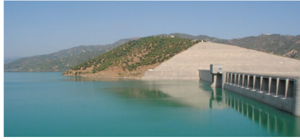
FIGURE 1.3: Koudiat Acerdoune Dam [11]
