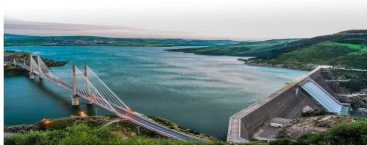
FIGURE 1.2: Beni Haroun Dam [11]
