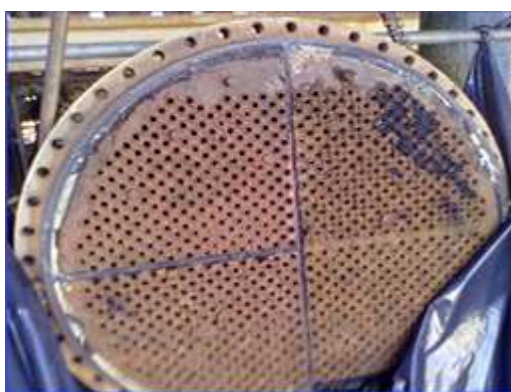
Figure III. 6: Isolation des tubes fuyards.
