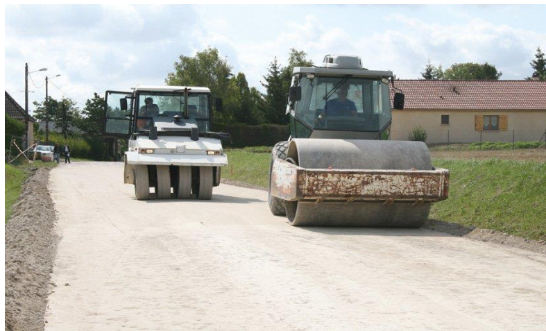
Figure II.1. Compactage de surface.
