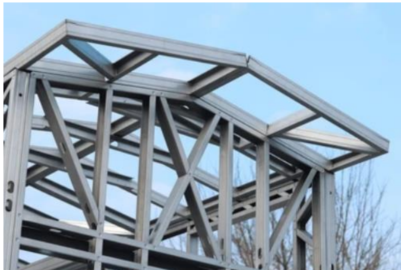
Figure I. 3: Structure en acier
