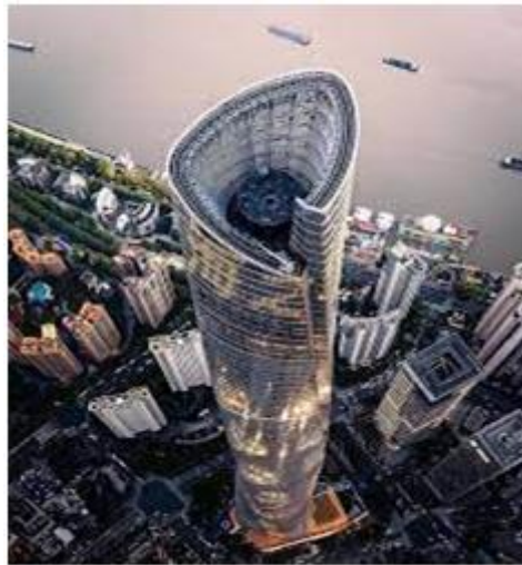
Figure IV. 2: La Shanghai Tower (Chine) [8].
