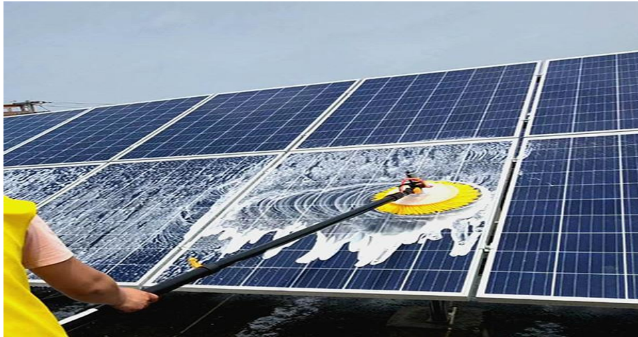
Figure III.1. Manual cleaning with water, brush and soap [52]
