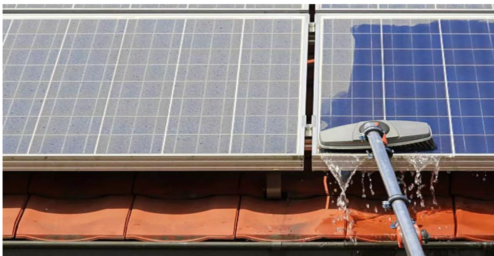
Figure III.2. Soap-less cleaning with deionized water and brushes [53]
