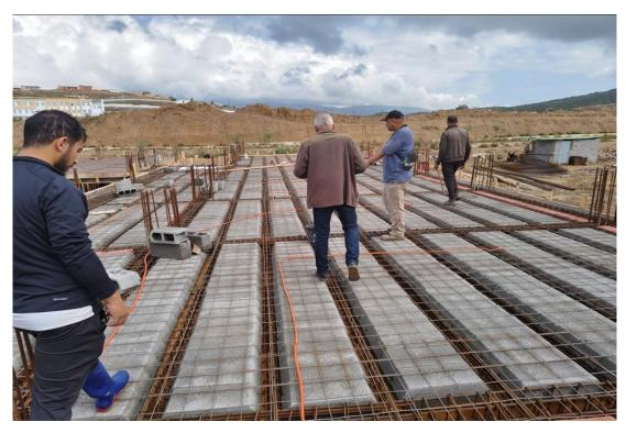
Figure 28 : Reinforcement and formwork for slab LEVEL+3.40 joint 3 Source: « DIB SALAH « company
