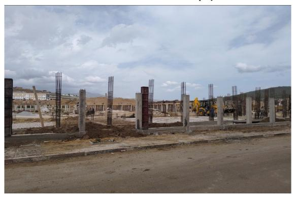
Figure 29 : Reinforcement and formwork for the columns at level +3.40 joint 6 Source: « DIB SALAH « company
