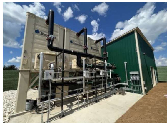
Figure III-13: Geothermal Heating and Cooling [Geogrid system]
