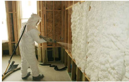
Figure III-20: high-density spray foam, thermal insulation
