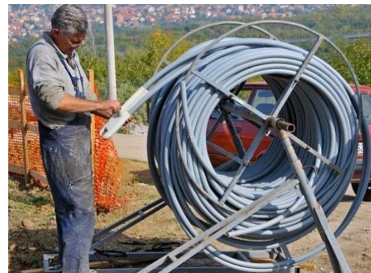
Figure III-18: REHAU RAUGEO™ PEXa double U-bend pipe loops),
