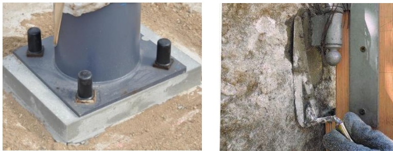
Fig 7.4: Wedging a steel frame post.
