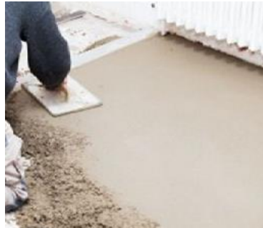
. Fig 7.3: Application of screed coating.
