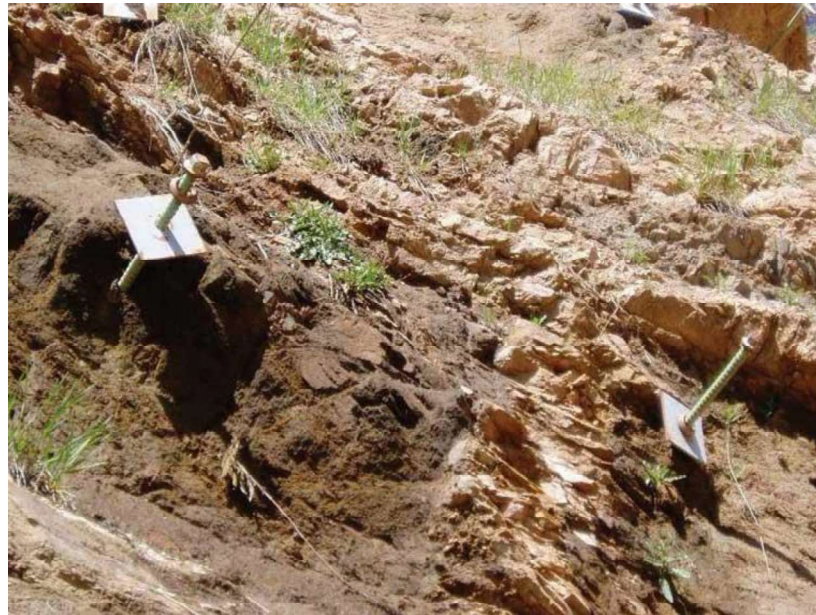
Figure III.31 Rock bolts installed in an area where the surrounding rock has eroded away, reducing the effectiveness of the bolts. [33]
