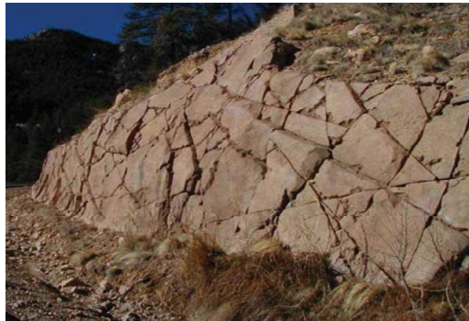
Figure III.36 Shotcrete can be used to protect a slope from erosion-and sculpted to mimic the natural rock face [33]
