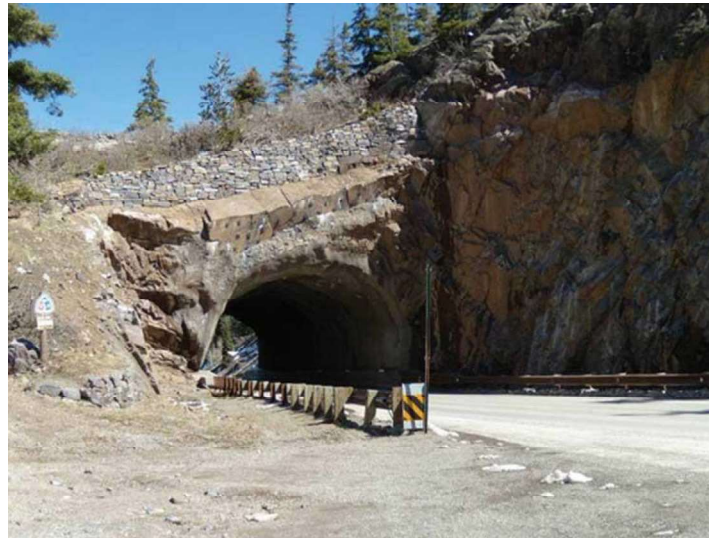
Figure III.37 Sculpted shotcrete used to stabilize a tunnel portal (the area directly below the dry-stack wall is the sculpted shotcrete). [33]
