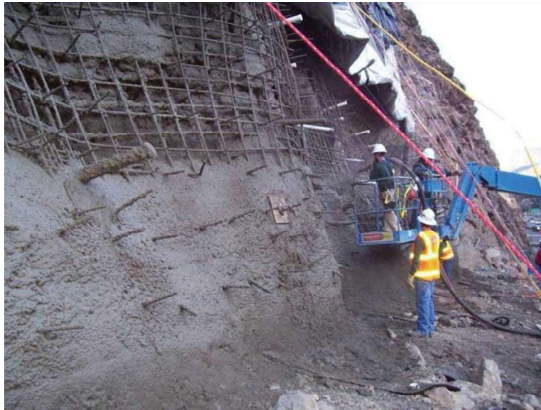
Figure III.38. Application of the first layer of structural shotcrete. .[33]
