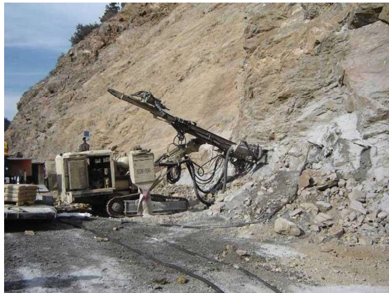
Figure III.32 Installation of rock bolts using a track drill. [33]
