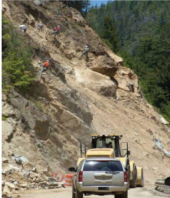
Figure III.26 Hand scalers removing loose material from a cut slope South Fork Smith River Road, California. [33]
