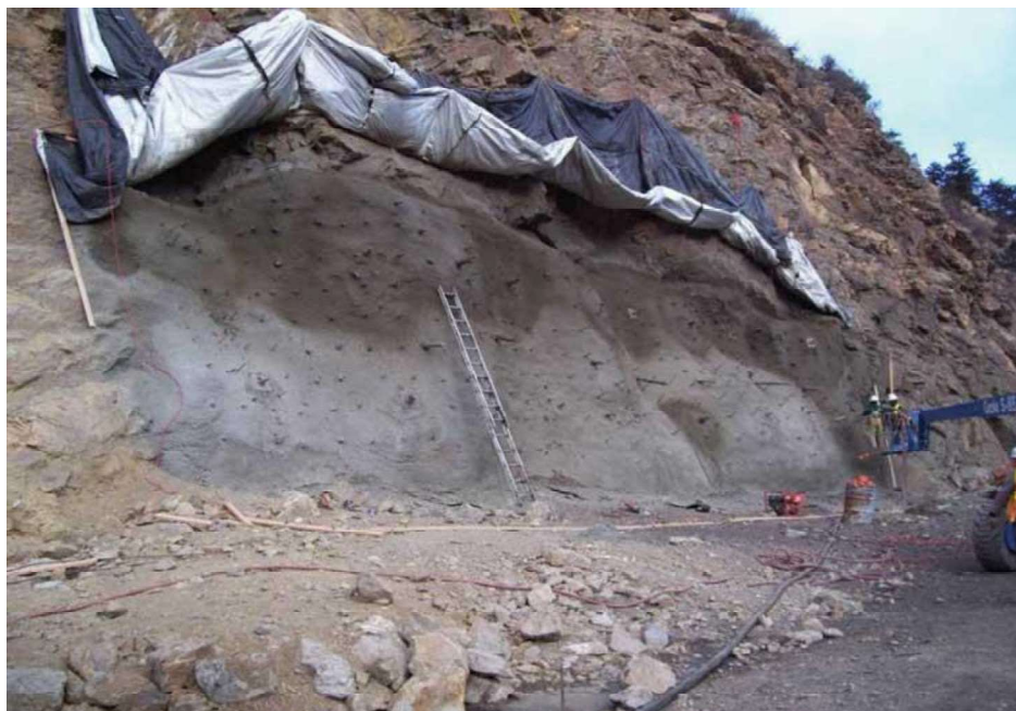
Figure III.39 Installation of the first layer of structural shotcrete [33]
