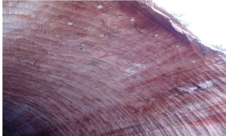
Figure III.30 Tunnel crest supported with dowels that have been covered with colored grout. [33]
