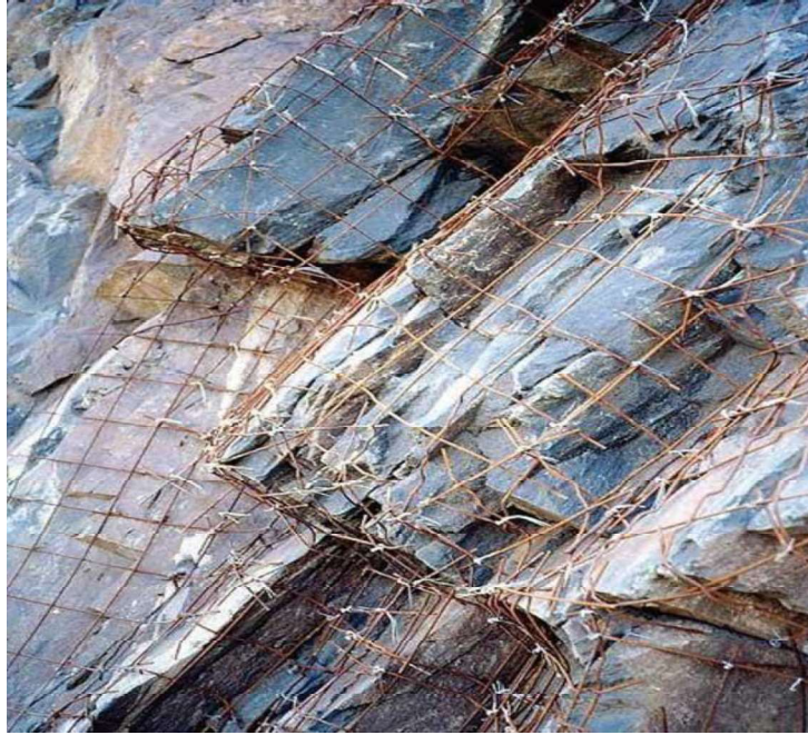
Figure III.35 Welded wire mesh can be attached to the rock face before shotcrete is applied.
