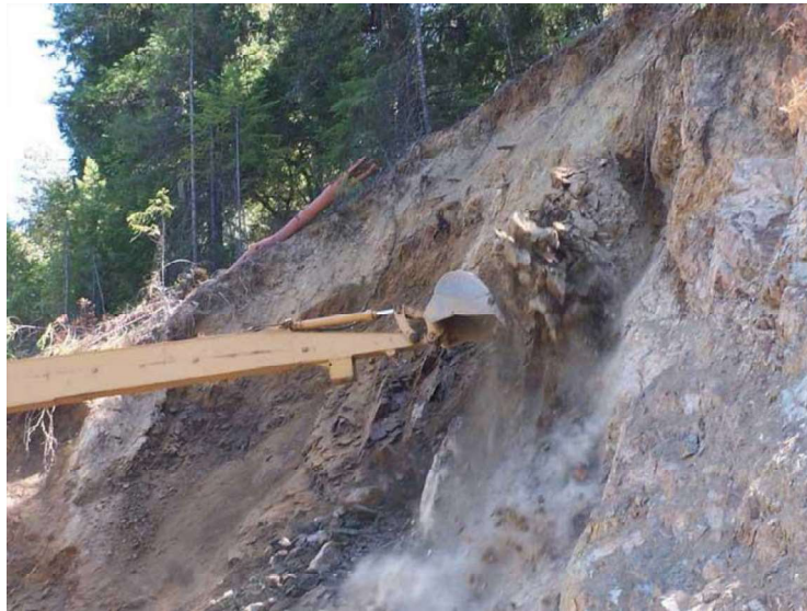
Figure III.27 Using a long-reach excavator for mechanical scaling. .[33]
