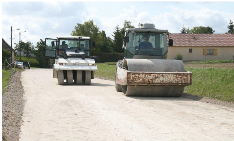
Figure II.1. Compactage de surface.
