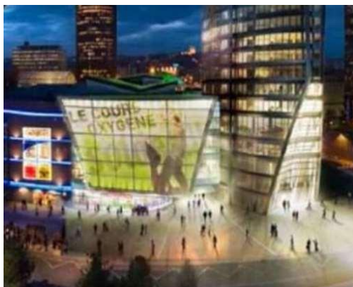
Figure 83 la façade principale
