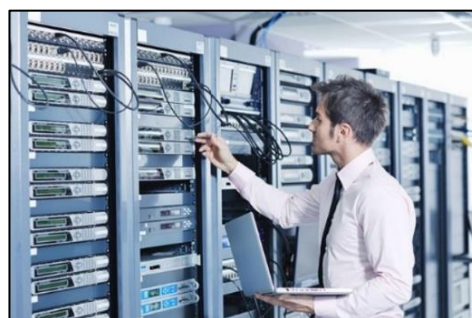
FIGURE 46: SALLE DE MAINTENANCE
