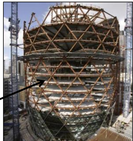
Figure 55: La structure Diagrid system Source : aedesign.files.wordpress.com
