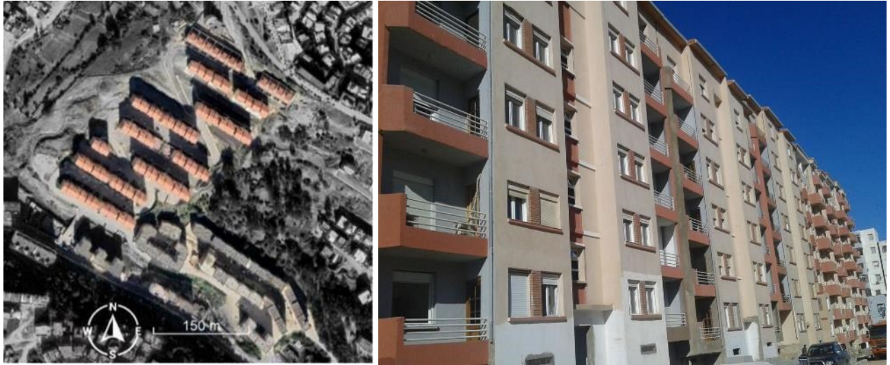
Figure V. 22. Aerial view of examples of promotional collective housing in Skikda: in Oued el wahch.
