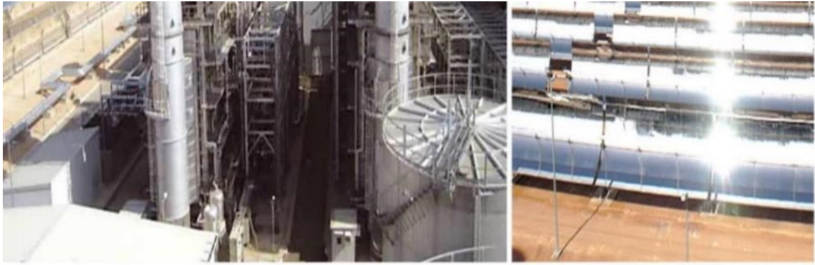
Figure III. 9. CSP station of Hassi R'mel.
