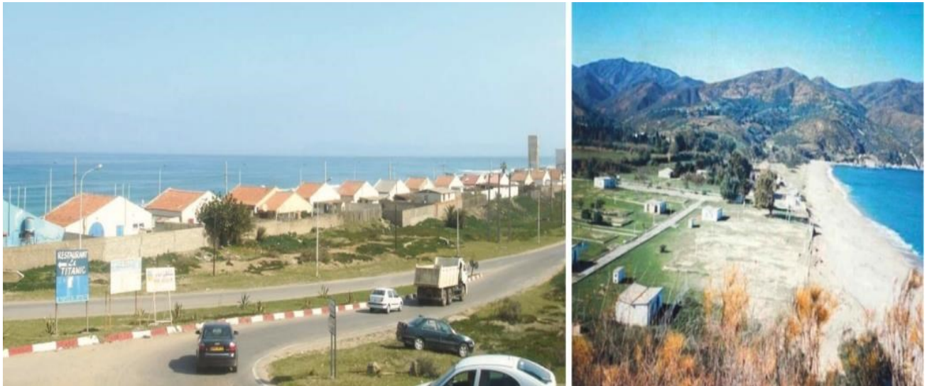
Figure V. 23. photographic shots of prefabricated chalets in Ben Mhidi's ZET and "La grande plage", Skikda.
