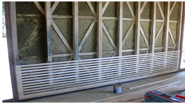
Figure I.4 Technique de torchis.
