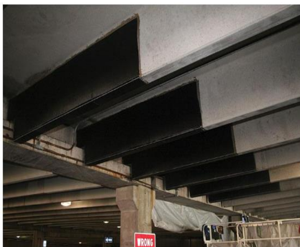
Figure II-10. Full wrapped RC beam by CFRP [41].
