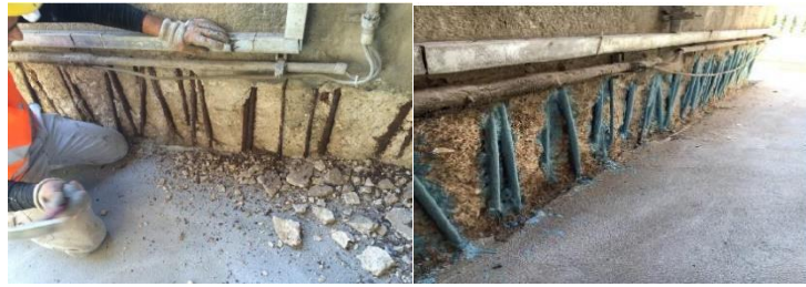
Figure I-14. Protective layer against corrosion [29].
