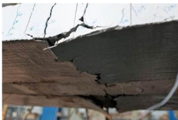
Figure II-13. FRP rupture in RC beam specimen [46].
