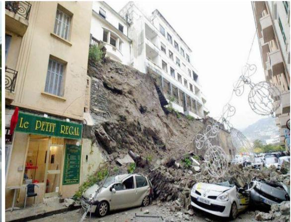
**Figure V.13** Surcharge (excessive nouvelle construction).
