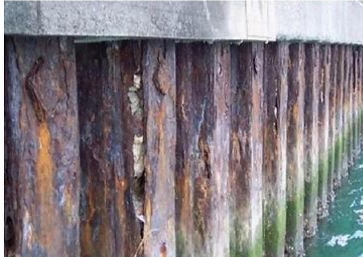
**Figure V.38** Corrosion de palplanches.
