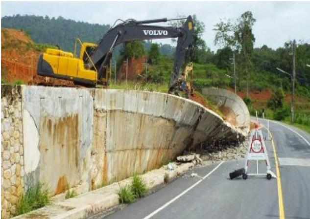
**Figure V.12** Surcharge excessive (engins + travaux).
