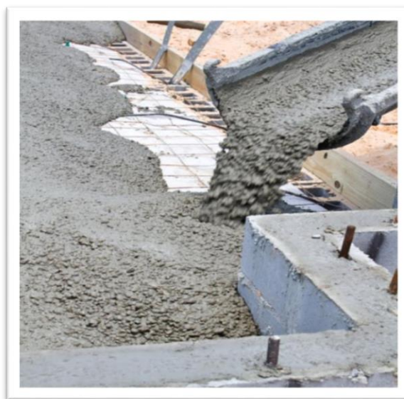
Figure I.3 : Application de béton fluide. [7]
