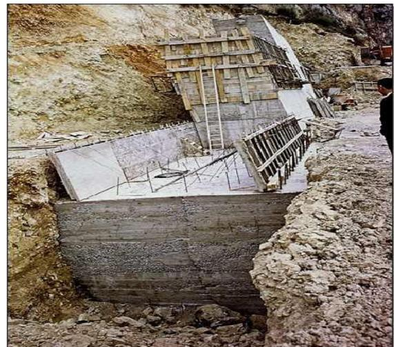
**Figure I.7 :** murs cantilever.
