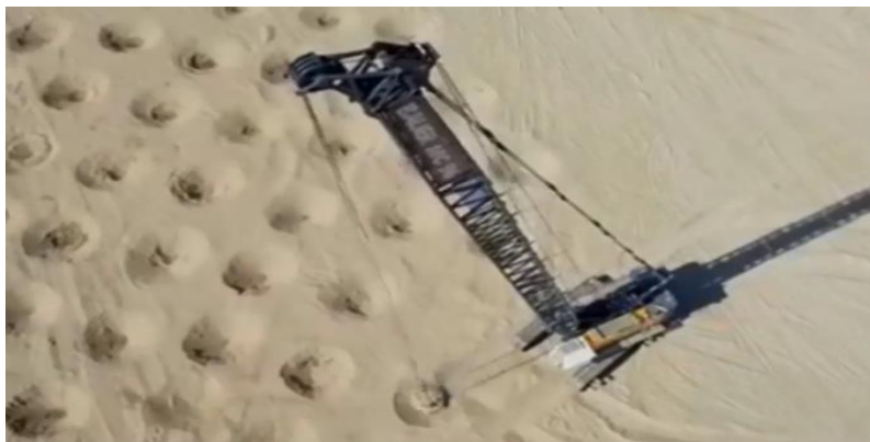
Figure I.17 Compactage dynamique
