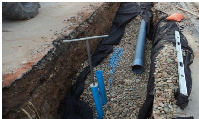
Figure II.2 Remblais courant (tranchée drainante)
