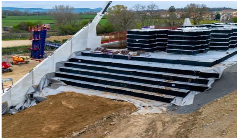
Figure II.11 Remblai en NIDAPLAST RA
