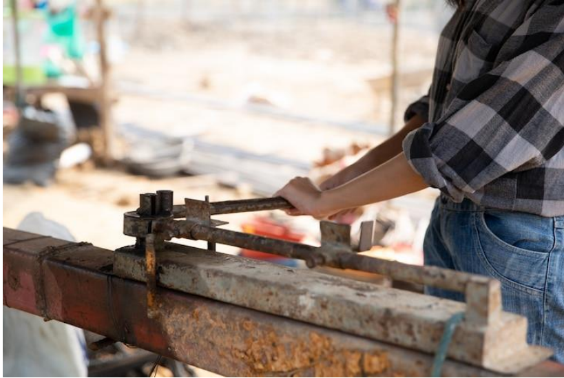
Figure I-7: manually rebar bending [15]
