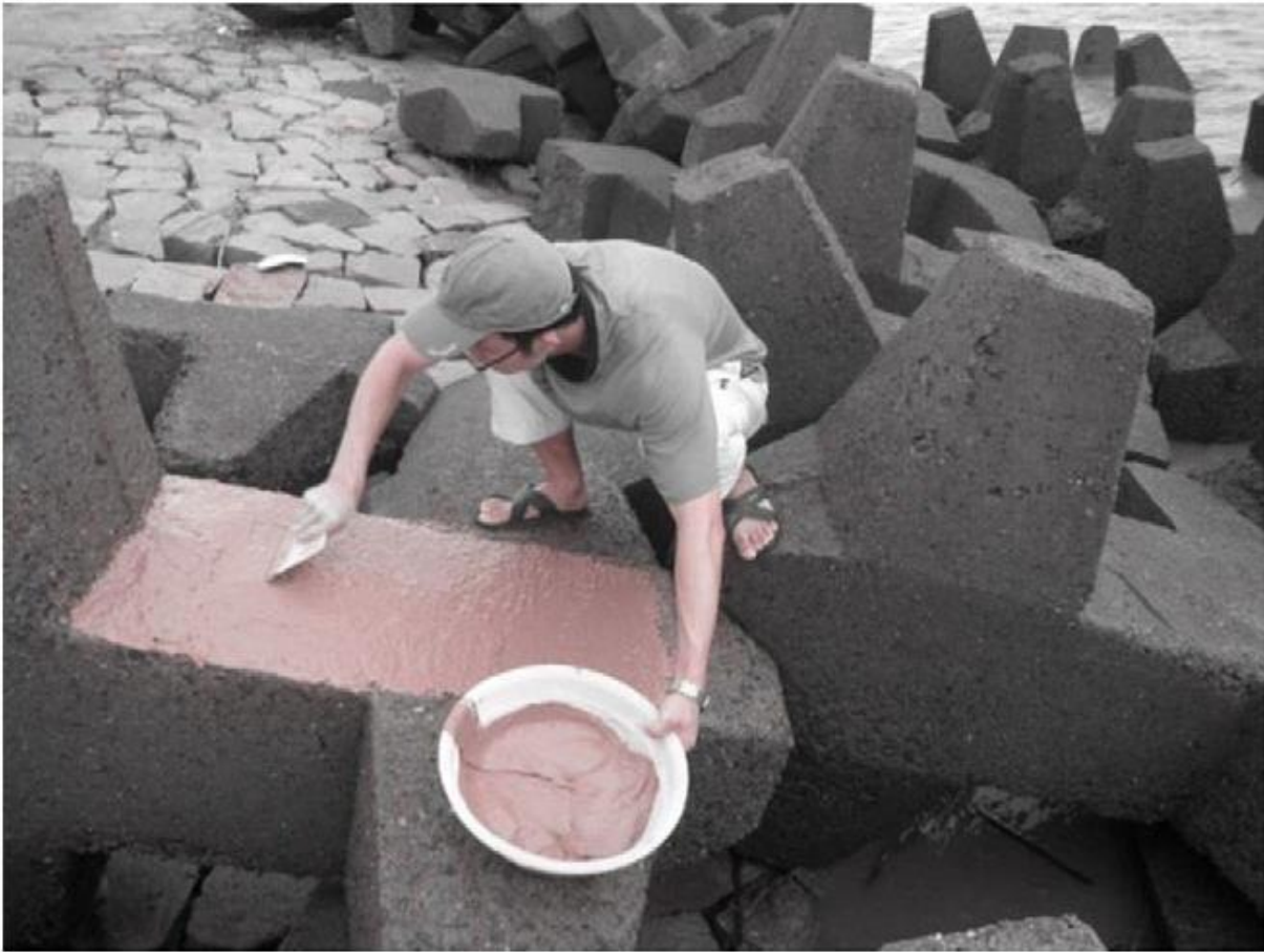
Fig 11: The use of geopolymer as anti-corrosive coating for marine
