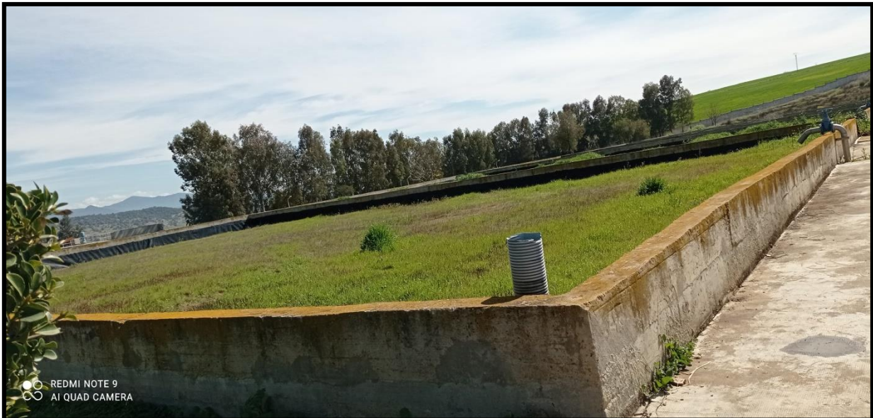
Figure 14 : Lits de séchage. (Yassad & Haiahem, 2022).
