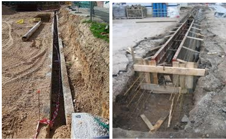
Figure I.6. Les murettes-guides [19].
