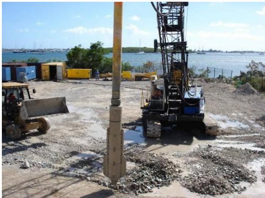
*Figure 14. Technique de vibrocompactage*
