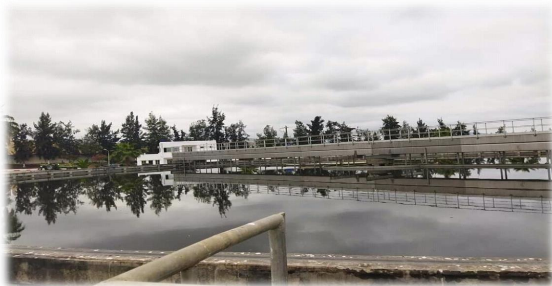
Figure II.7: Clarificateur (STEP Guelma 2021).
