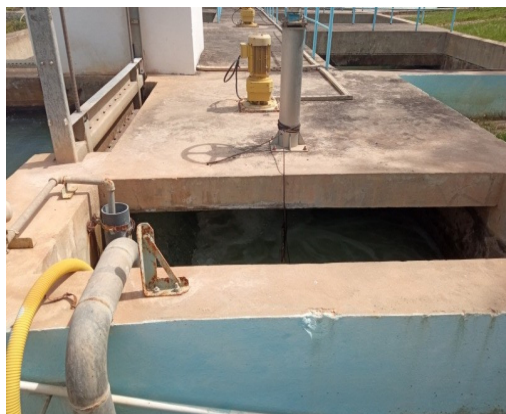
Figure I.III.3: Bassin de coagulation (agitation rapide).
