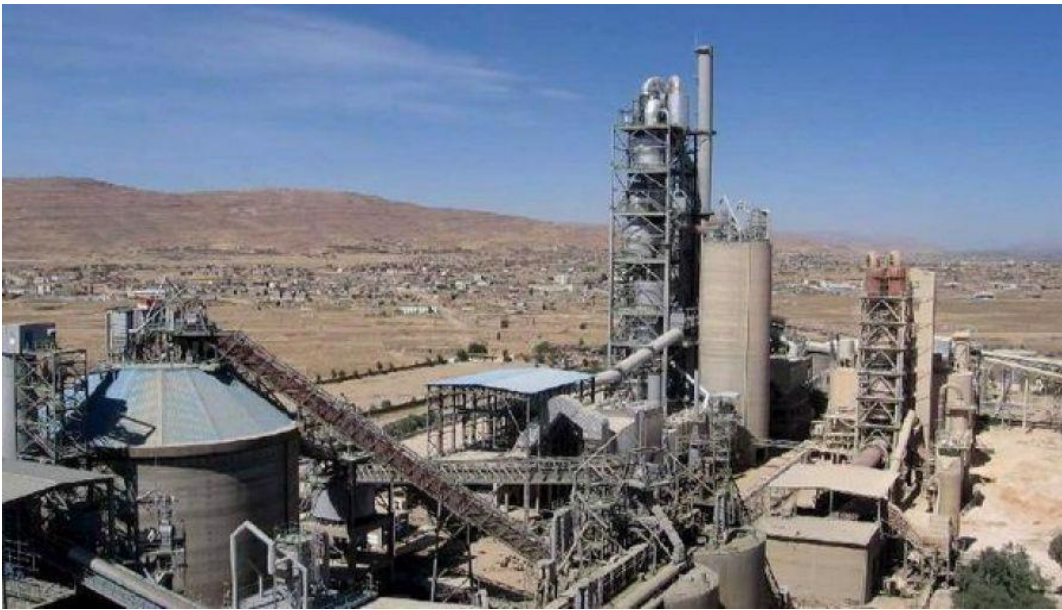
Figure 1: Cimenterie de Hadjar Soud (SCHS)
