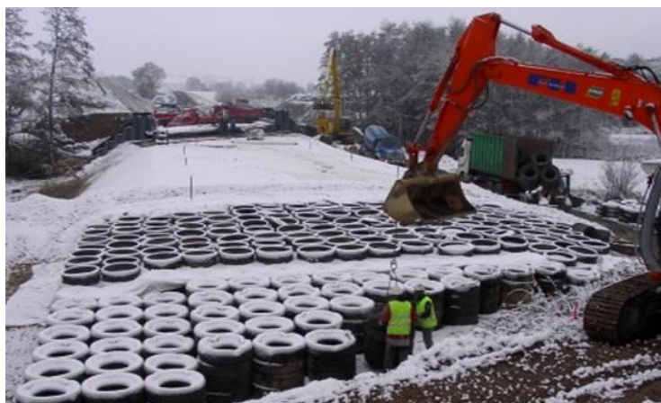
Figure III.9 La technique pneusol [7]
