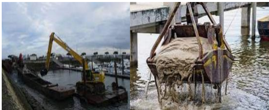
Figure. III.15 Dragage des sédiments [20]
