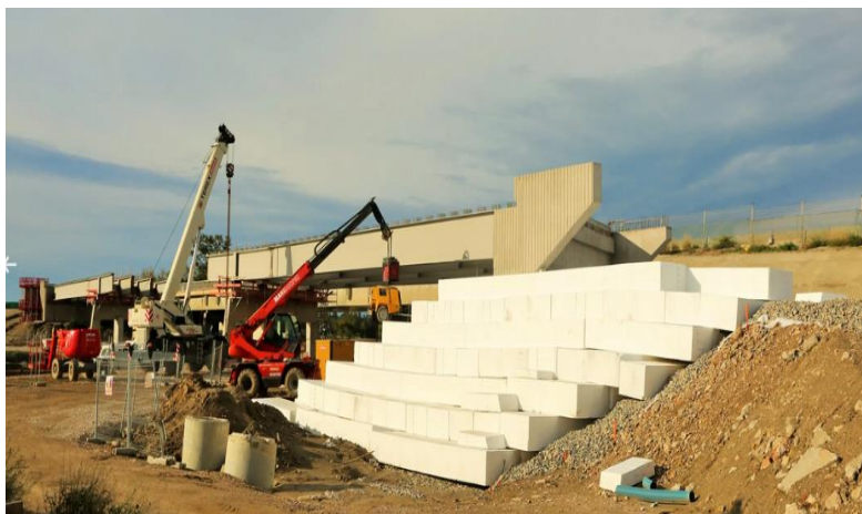
Figure II.11 Remblai allégé polystyrène
