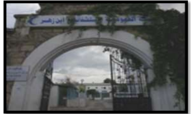
Figure 61:hôpital Ibn Zohr
