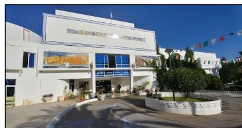
Figure 45: facade du complexe
