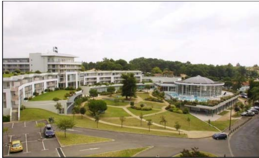
Figure 45: Volume de station de Caliceo. Source : www.allo-thalasso.com
