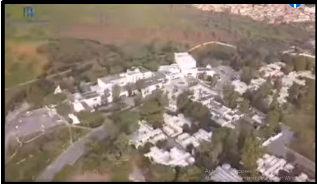
Figure 26: complexe chellala . Source : personnel .
