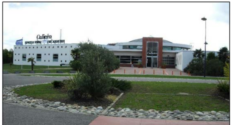
Figure 39: Station Thermal Caliceo. Source : httpswww.monnuage.frpoint
