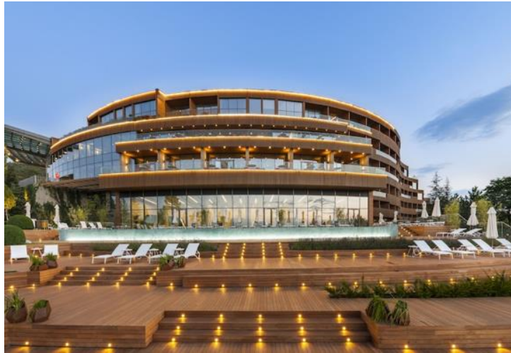
Figure 60 :la façade principale de tasigo
