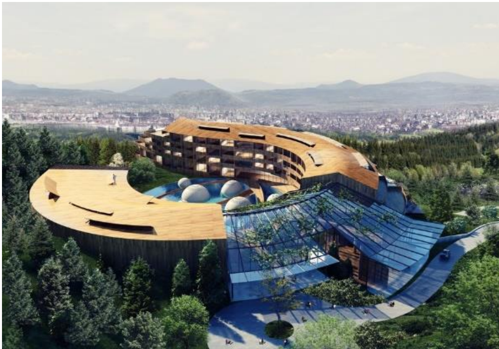
Figure 51 :le volume de centre thermal Eskisehir
