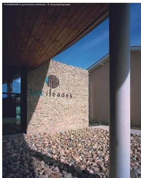
FIGURE 71 FIGURE 72 :UTILISATION DE PIERRE
