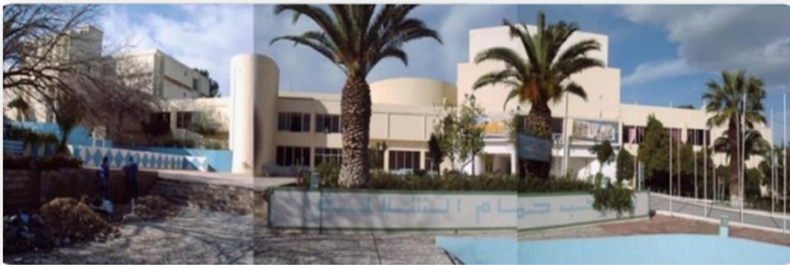
Figure 76 :le complexe thermal hammam challala
