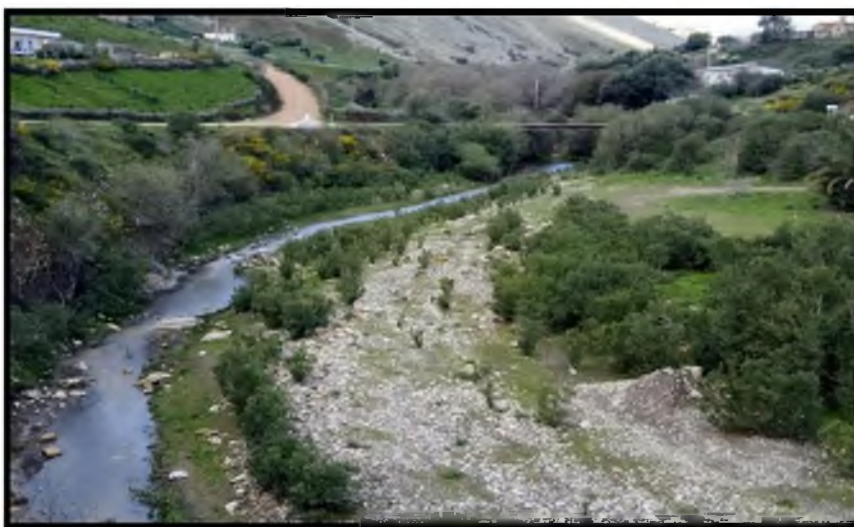
Photo 15 : Station Hlia amont (2)
